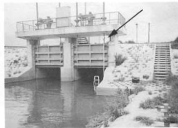
Open angle control of the river gate (The PL is in the stilling tube)
